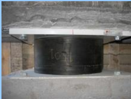
33 bearing isolators FIP SI-N 400/108
